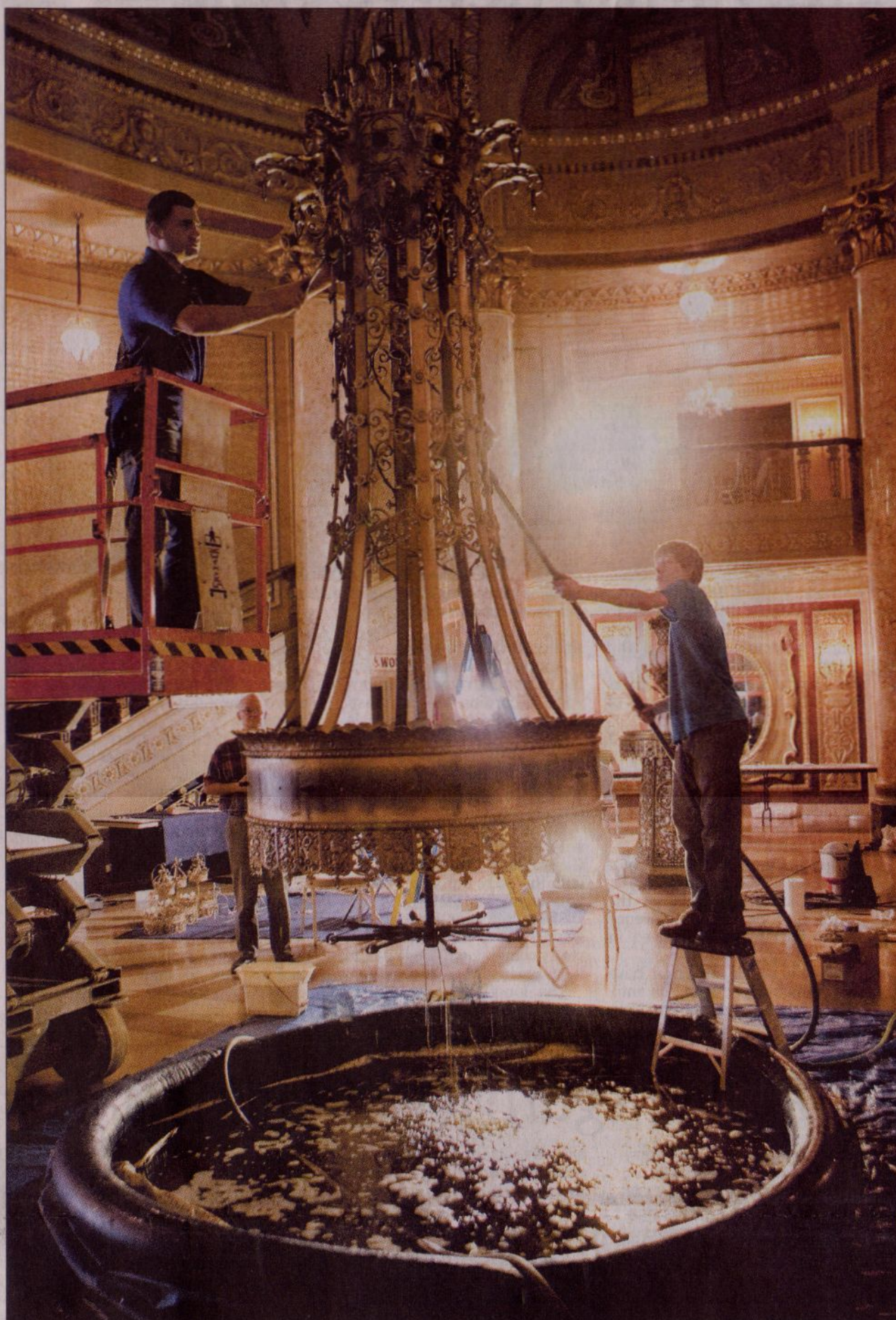
Lukasz Marona, left, and Alex Janko clean the brass on the main fixture of the Duchess, the 22-foot-tall, 2.5-ton chandelier that hangs in the rotunda of the Rialto Square Theatre. DAVID PIERINI/TRIBUNE PHOTOS
